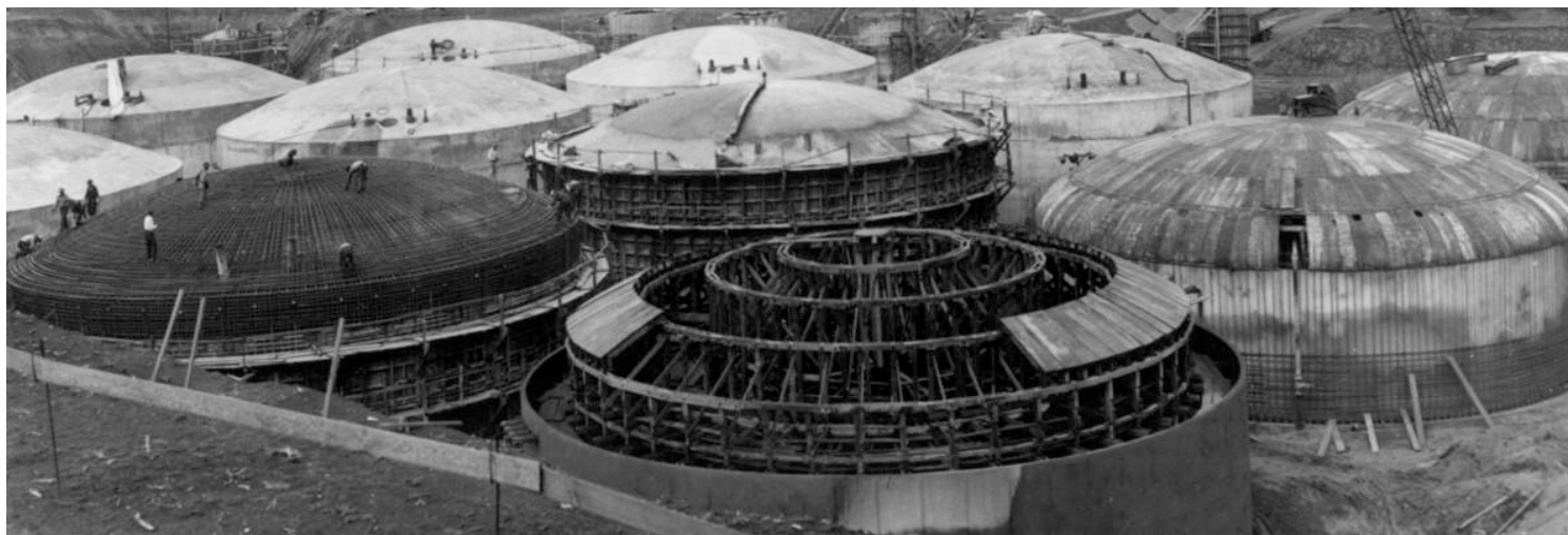
Construction of the original storage tanks at the Hanford Site. These 530,000-gallon capacity underground storage tanks were built between 1943 and 1944, and put into service in 1945 to store radioactive sludge. NETL is modeling part of the process to clean up this radioactive waste for permanent storage.
